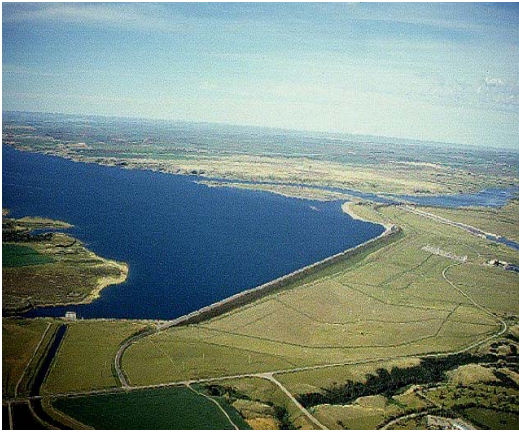
Figure 7. Gardiner Dam, the world's 17th largest dam was constructed by PFRA in 1968. It supplies drinking water to about 50% of Saskatchewan, enhances aquatic biodiversity, and is used for irrigation, hydroelectricity, and recreation.
