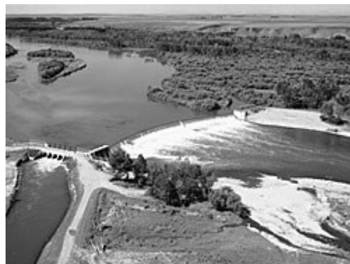
Carseland Weir is the main diversion structure delivering water to the Bow River Project
