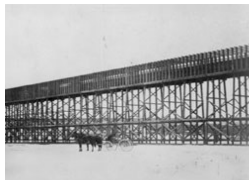
"Mile-Long Flume", part of the Bow River Project
