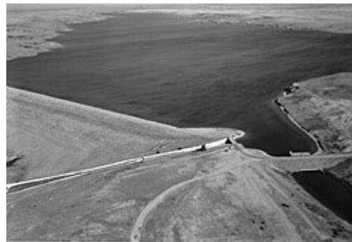
The Travers Dam and reservoir one of the main water storage projects for the Bow River
